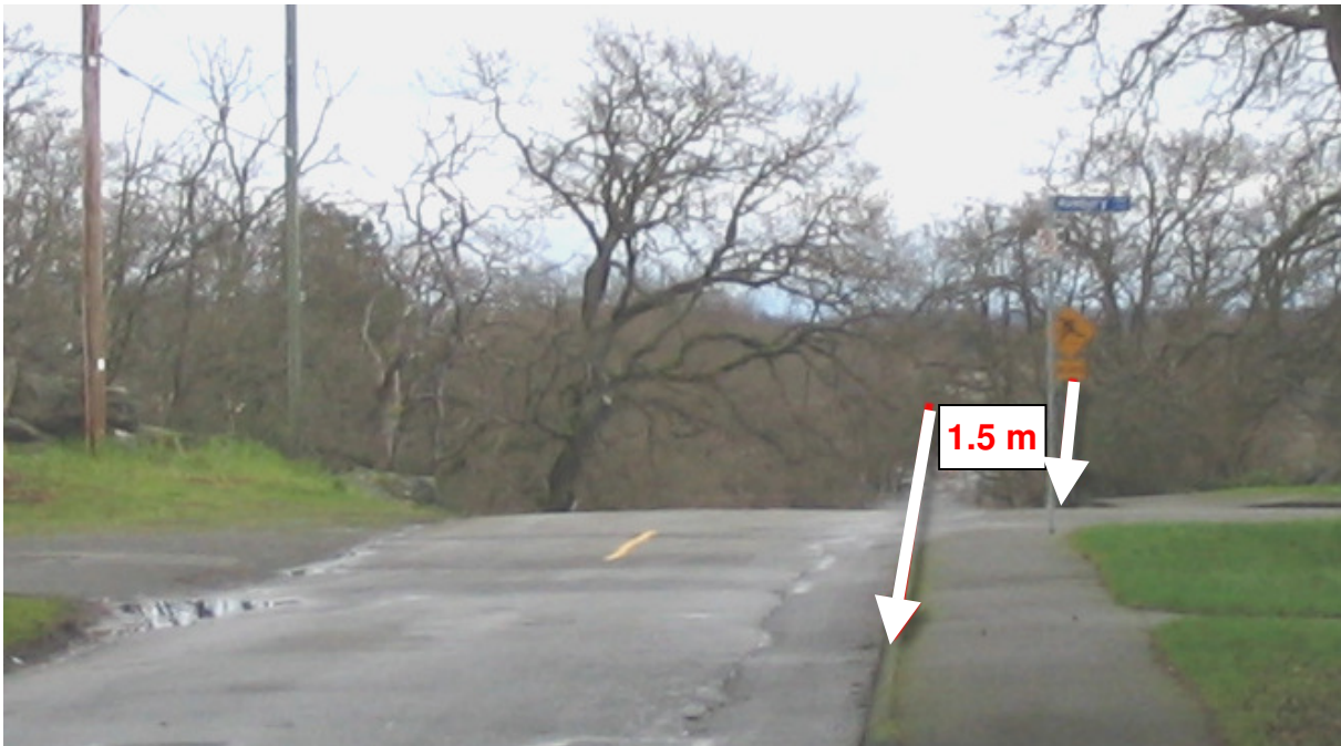
Photo 3 - 1.5 m curb setback occurring across the Avebury intersection at the crest of Ryan Hill.
