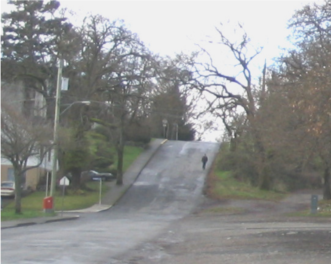
Photo 5 - Ryan Hill; note pedestrian walking on the north side pavement
