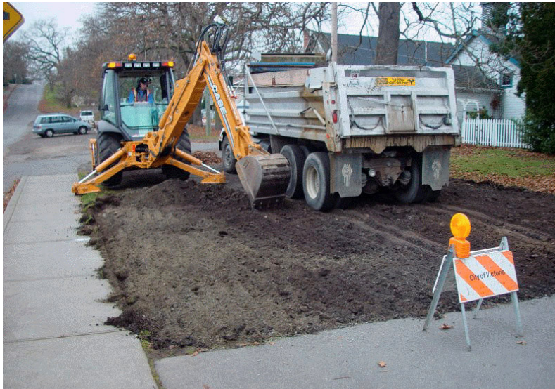
Digging up the parking lot
