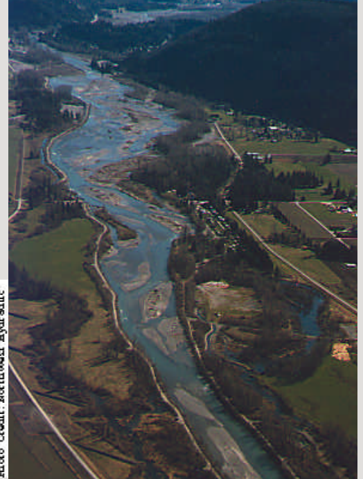
Photo Credit: NorthWest Hydraulic
